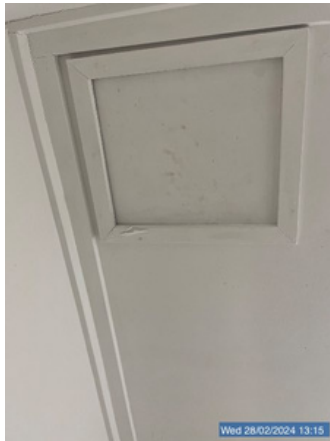
Ensuite: Ceiling/light fittings (photo 1 of 3)
