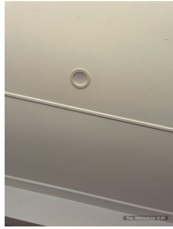
Kitchen: Ceiling/light fittings (photo 2 of 6)
