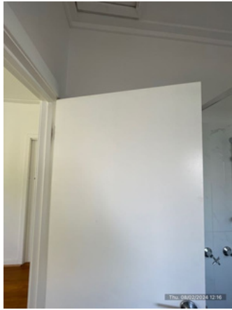
Ensuite: Doors/doorway frames (photo 1 of 22)
