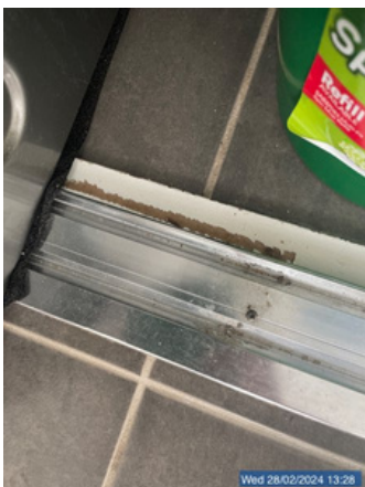
Laundry: Floor tiles/floor coverings (photo 1 of 2)
