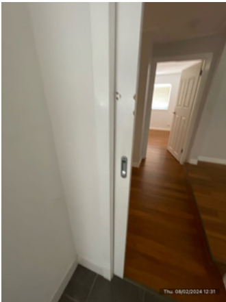
I Bathroom: Doors/doorway frames (photo 3 of 16)
