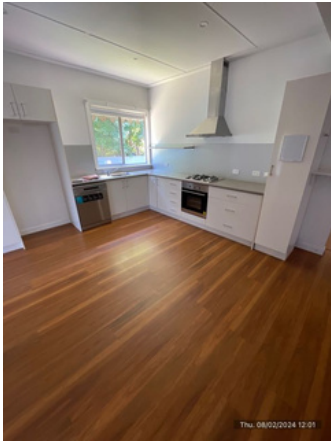
Kitchen: Overall (photo 1 of 1)
