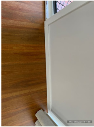
Lounge Room: Skirting boards (photo 1 of 8)
