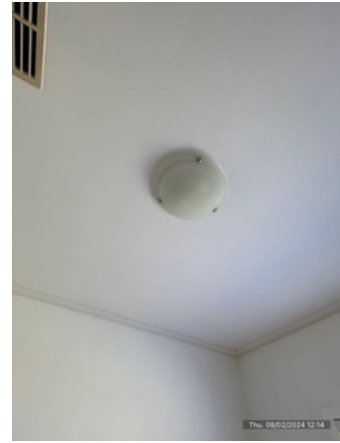
Bedroom 1: Ceiling/light fittings (photo 1 of 4)
