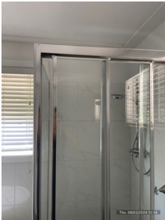
I Bathroom: Shower/screen/taps (photo 3 of 9)
